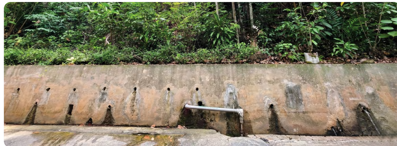
Spring water recovery system at AEON Mall Alpha Angle, redirecting natural flow from the adjacent jungle and collected for non-potable cleaning operations.
